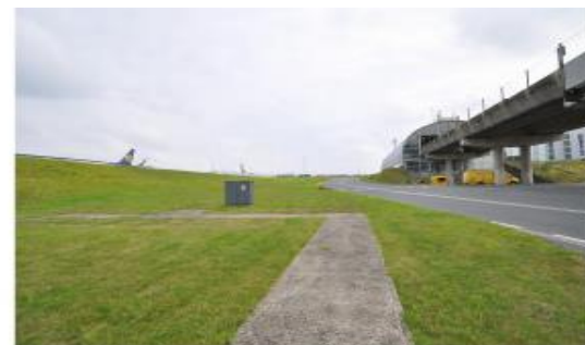
2 - VIEW OF TTS MAINTENANCE AND PROPOSED SITE OF PLANT ENCLOSURE
