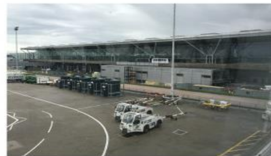
3 - VIEW OF TERMINAL FROM APRON 1 AND BUS-GATE BUILDING
