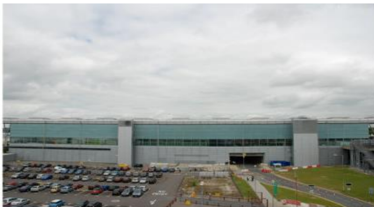
1 - VIEW OF WESTERN FACADE OF TERMINAL
